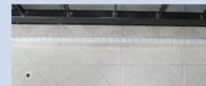
Holes are drilled at a distance of 50 cm.
