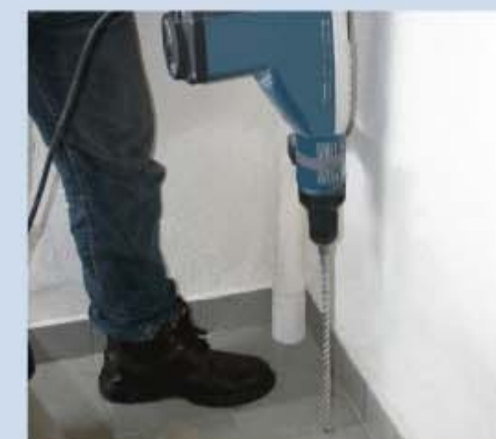
Concrete slabs have to be drilled.
